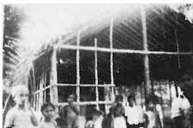
The Sunday School shed under construction at Kanjiran Clurrai, Alleppey
